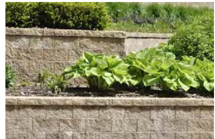
Figure 2.52 Multiple retaining walls with planted terraces
