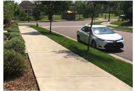
Figure 2.43 Parallel parking along internal streets
