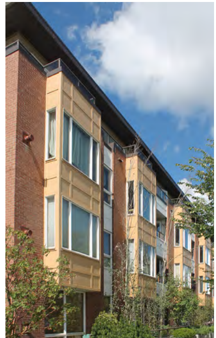
Figure 2.2 Example of Multiple-Family building
