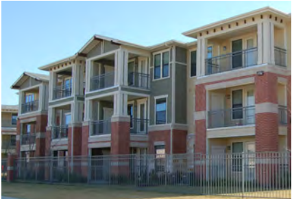
Figure 2.110 Horizontal massing defined by material changes
