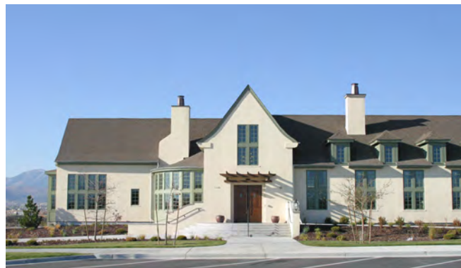
Figure 2.106 Example of club house Amenity Building
