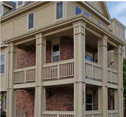
Figure 2.126 High-quality and well-designed wrapping Porch and Balcony
