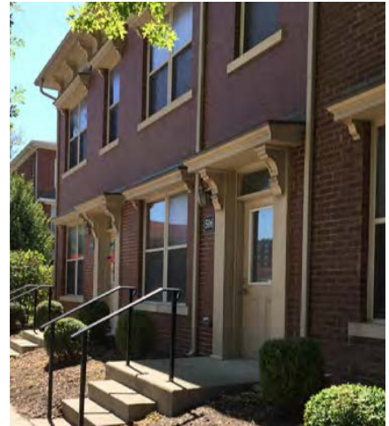
Figure 2.69 Example of a high-quality townhouse development
