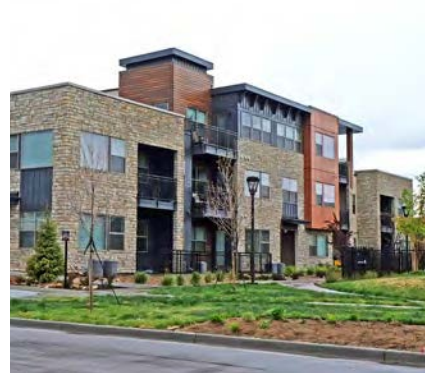
Figure 2.89 Example of Walk-Up Multiple-Family Building
