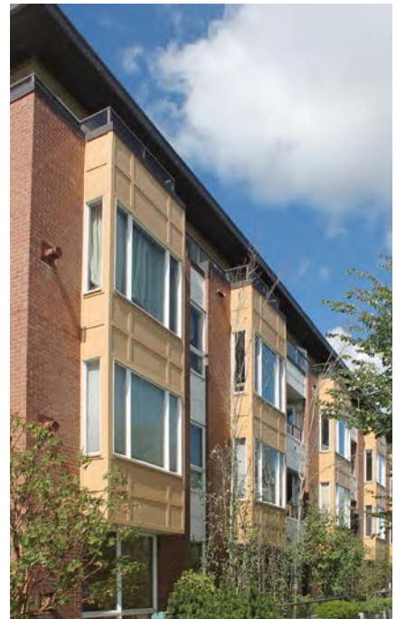
Figure 2.2 Example of Multiple-Family building
