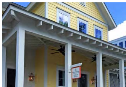
Figure 2.128 Simple Eave Overhang
