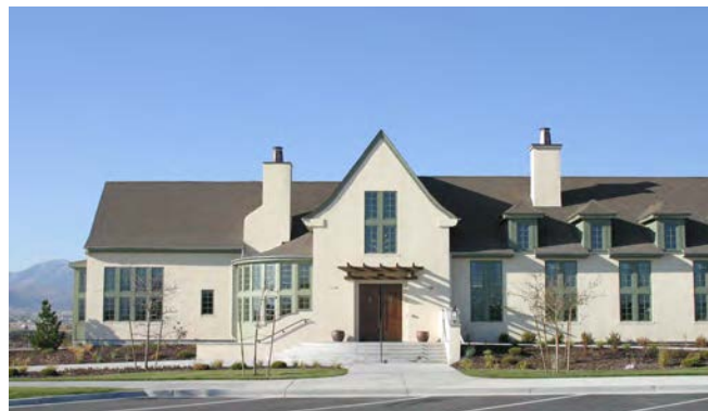
Figure 2.106 Example of club house Amenity Building
