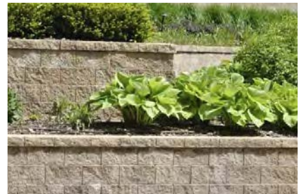
Figure 2.52 Multiple retaining walls with planted terraces
