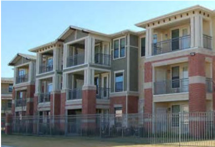
Figure 2.110 Horizontal massing defined by material changes
