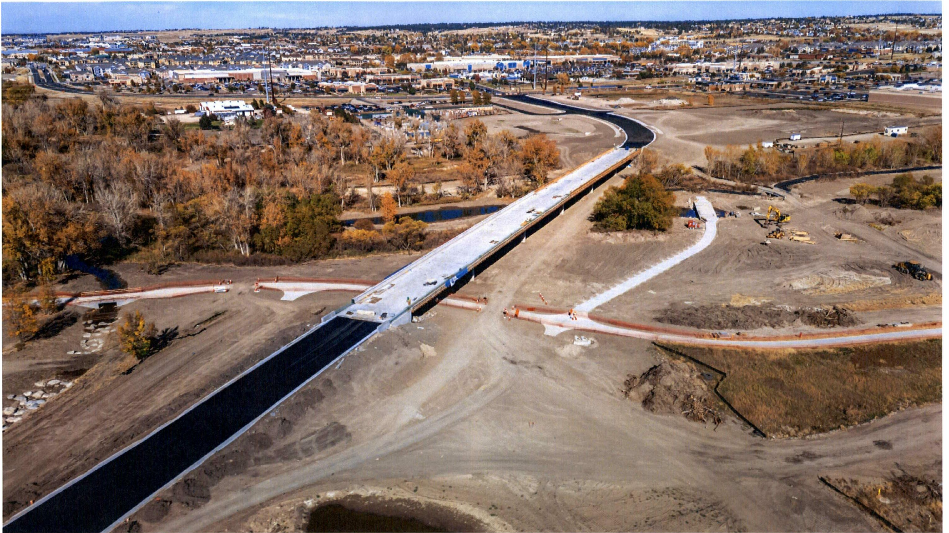
Dransfeldt Road Extension
