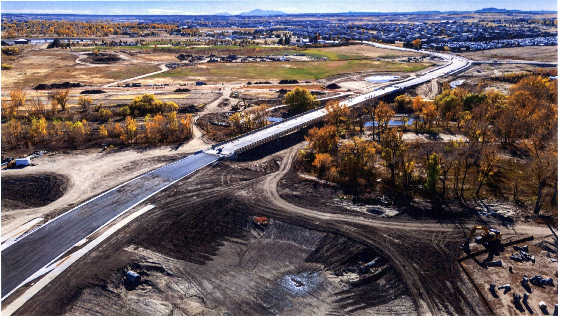
Dransfeldt Road Extension
