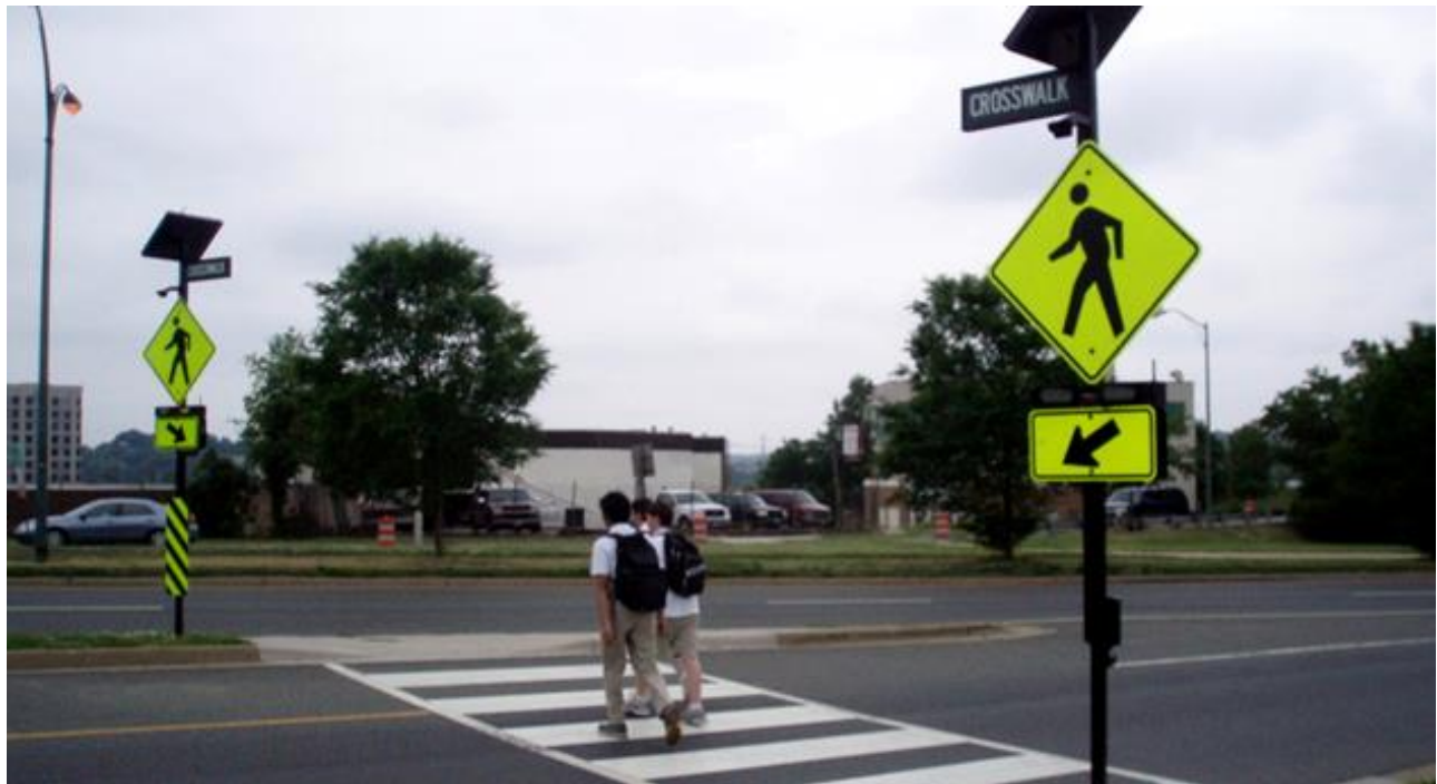
Figure 25: Rectangular Rapid Flash Beacons (RRFBs)
