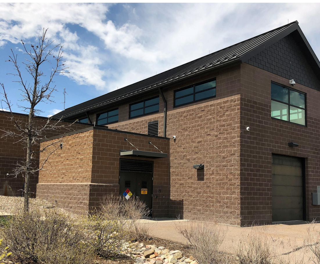
REGIONAL WELL HOUSE
