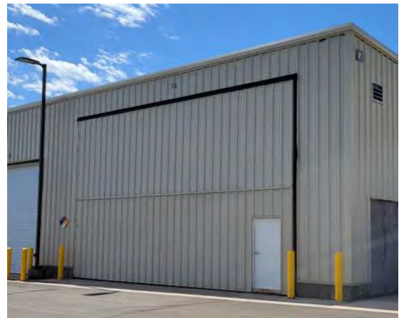
D2.3 Vertical lift bi-fold door
