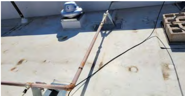
D3.1 Roof - TPO Membrane
