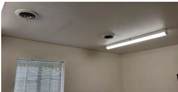
E2.1 Gypsum Board Walls
