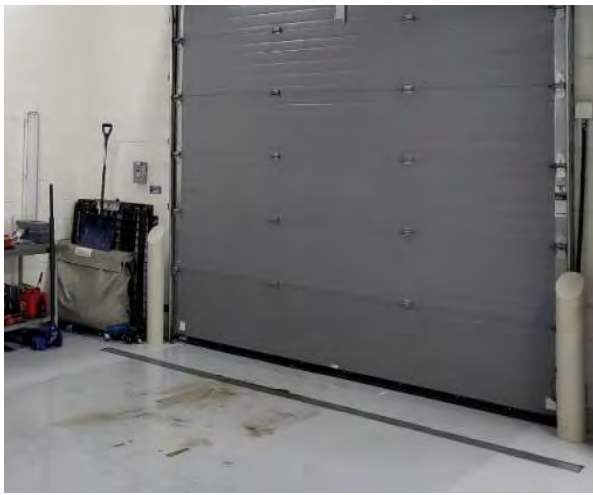
F7.1 Trench Drain To Sand/Oil Interceptor
