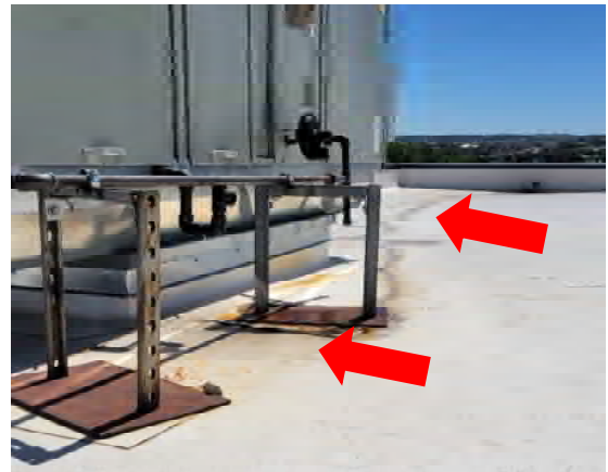
D1.6 Condensate Surface Drainage
