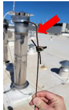
D1.6 Flue Stabilization - Rusted Cables
