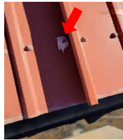
D1.2 Standing Seam Metal - Caulked Exposed Fastener
