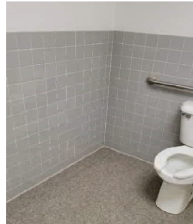
E2.2 Tile Walls - Restrooms
