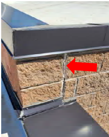
D1.3 Masonry Joint Sealant
