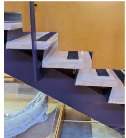
E7.1 Stairs & Railings - Stone
