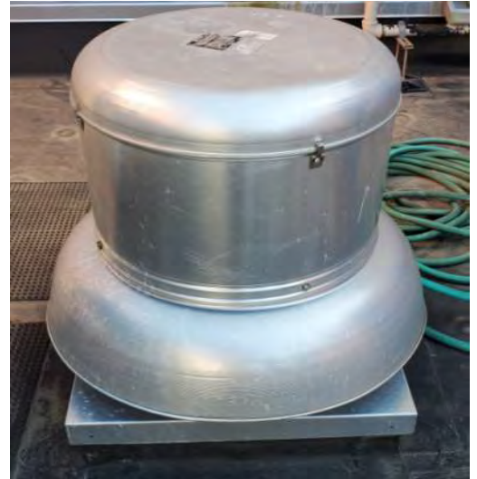
F12.1 Typical roof mounted exhaust fan.
