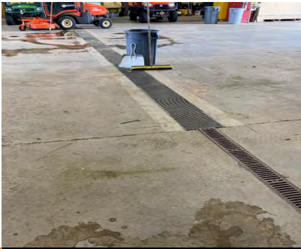
F7.1 Trench Drain To Sand/Oil Interceptor
