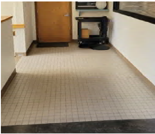
E1.2 Floor Tile - Entry
