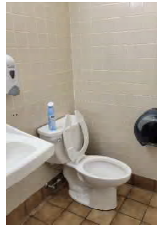
E2.3 Tile Walls - Restrooms
