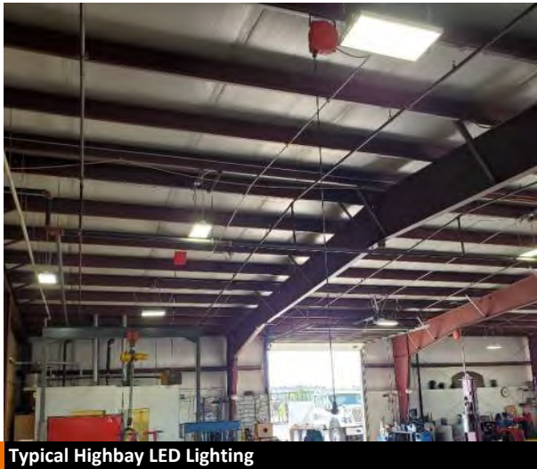
G2.1 Typical Highbay LED Lighting
