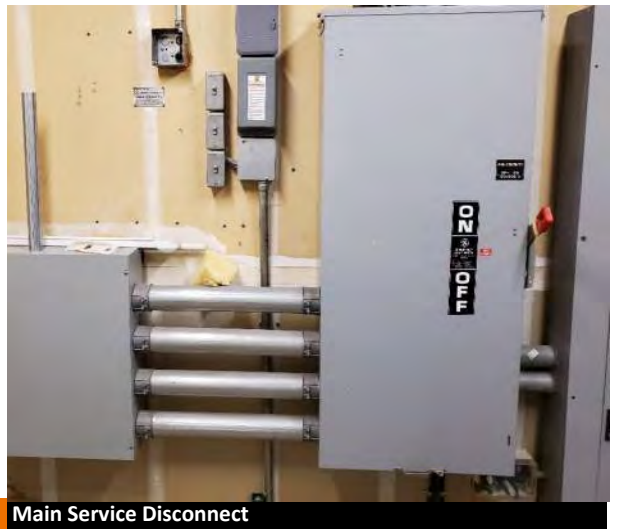
G7.1 Typical Disconnect Connection to Roof Top Unit
