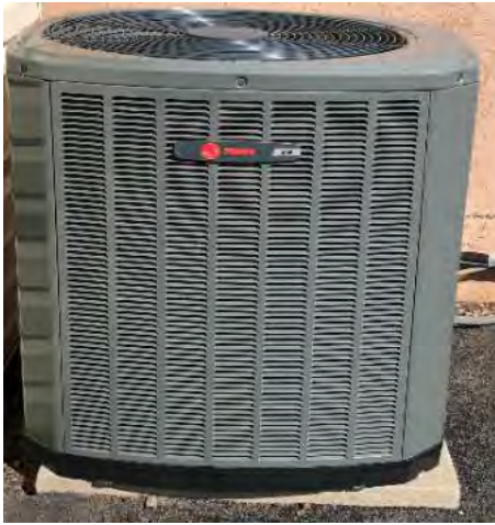
F10.1 Trane split system air conditioner.
