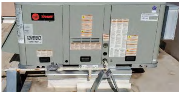
F9.1 Typical gas-fired rooftop unit.
