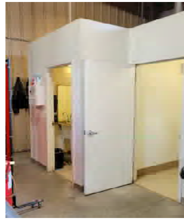
E2.3 Gypsum Board Walls
