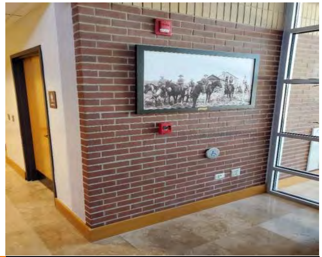
G6.1 Typical Annunciation Device - Horn/Strobe and Pull Station
