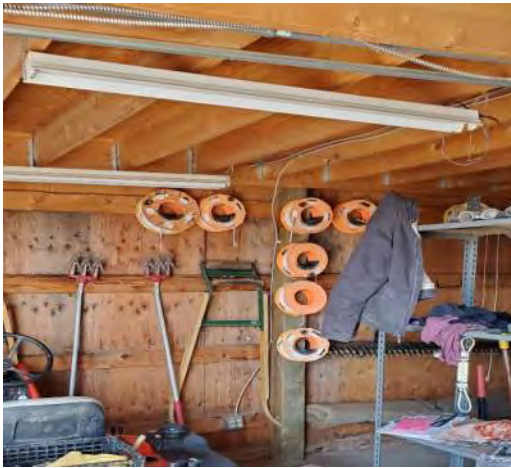
G2.1 Typical 1'x4' Fluorescent Strip Fixture
