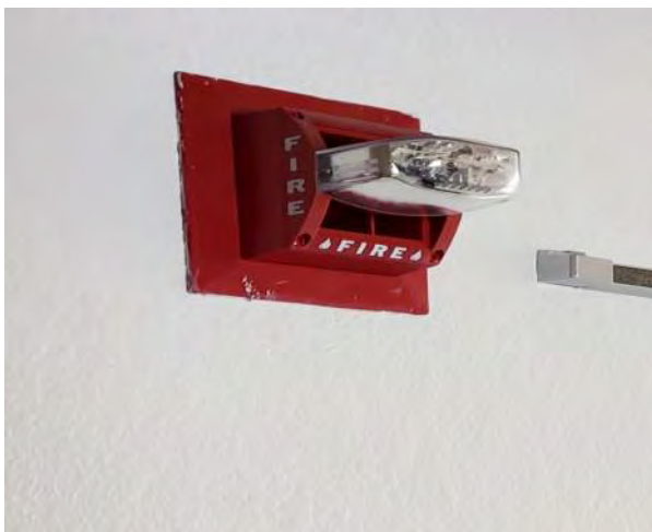
G6.1 Typical Annunciation Device - Horn/Strobe
