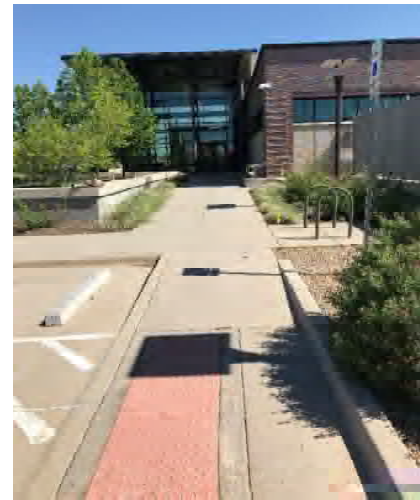
B4.1 West Entry - building access meets standards and in good repair
