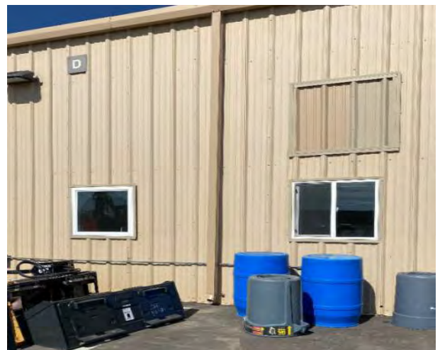
F4.1 Rain Gutters With Downspouts
