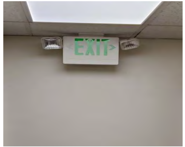
G4.1 Typical Exit/Dual Lamp Egress Fixture
