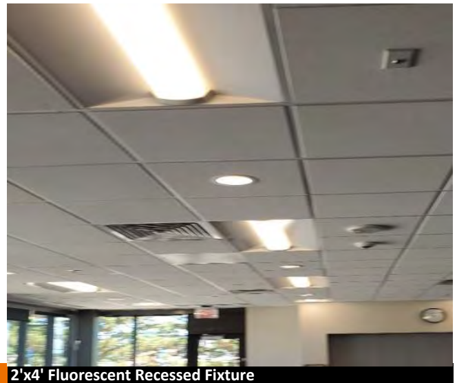
G2.1 2'x4' Fluorescent Recessed Fixture
