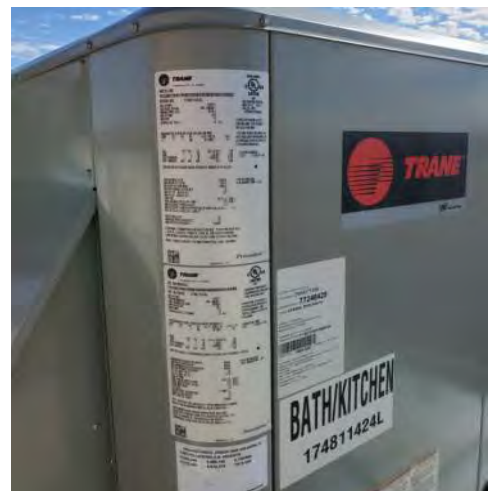
F10.1 Typical direct expansion (dx) rooftop unit.
