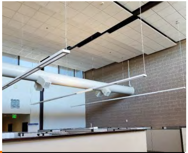
G2.1 Fluorescent Pendant Mount Linear Strip Fixtures
