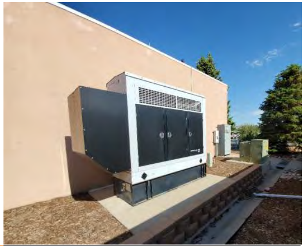
G5.1 Diesel Stand-by Generator
