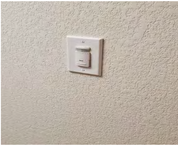
G1.1 Typical Wall Mount Occupancy Sensor
