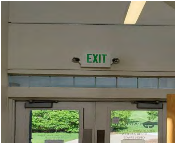
G4.1 Typical Battery Back-up Egress Lighting
