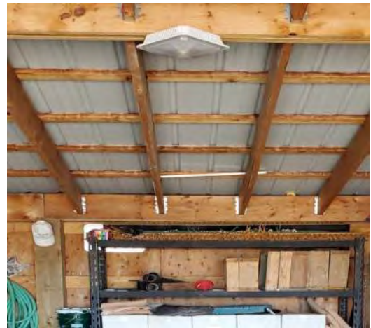
G2.1 Typical Surface Mount LED fixture
