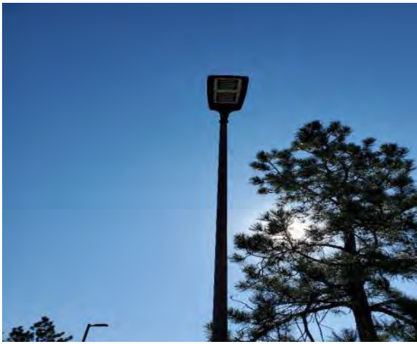
G3.1 LED Pole Mount Fixture
