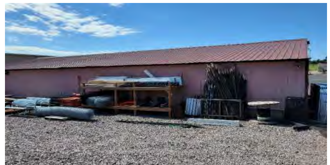
D6.1 Standing Seam Metal Roof
