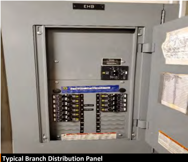
G8.1 Typical Branch Distribution Panel
