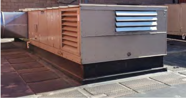
F11.1 Typical Mcquay rooftop unit outside air intake.
