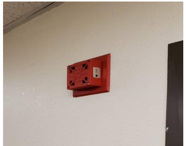
G6.1 Typical Annunciation Device - Horn
