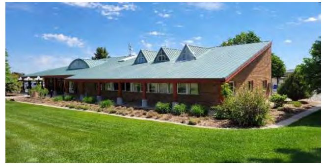
D6.1 Roof - Standing Seam Metal
