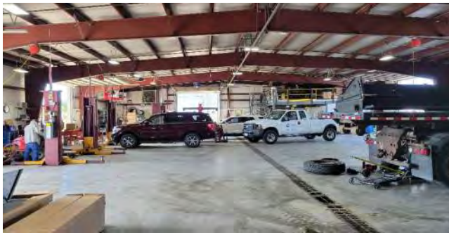
E3.1 Exposed Structure Ceiling
