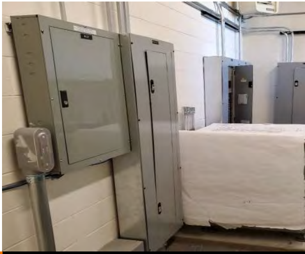
G8.1 Typical Siemens Branch Distribution Panelboard
