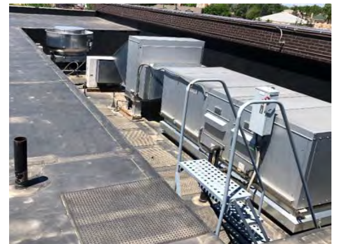
F12.1 Kitchen exhaust and make up air.
