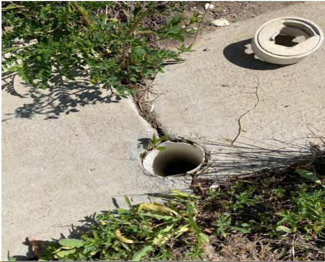
E4.1 Existing Potential Storm To Be Verified for Rain Gutters
