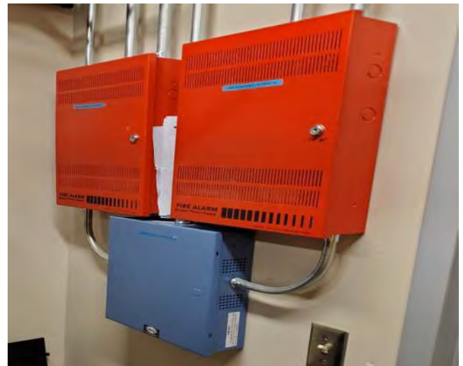
G6.1 Addressable Fire Alarm Power Supplies
