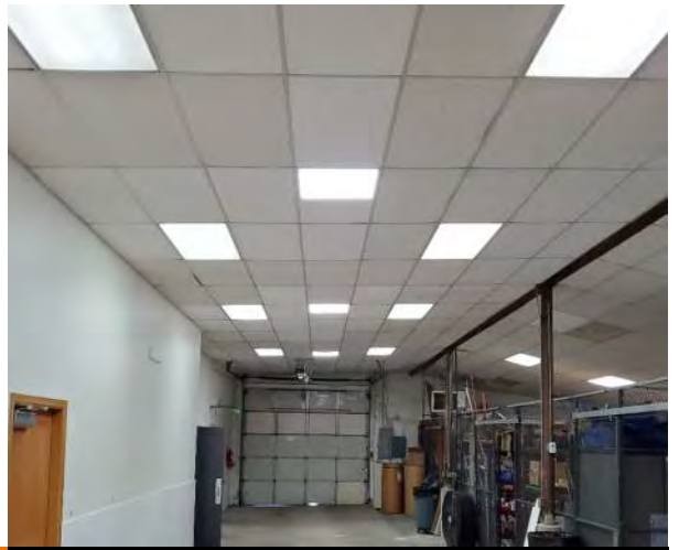
G2.1 LED 2'x4' Fixtures in Storage Area
