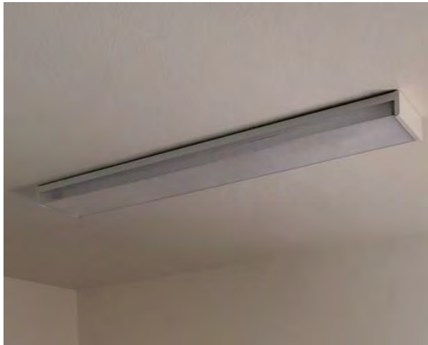
G2.1 Typical Linear Fluorescent Strip Fixture
