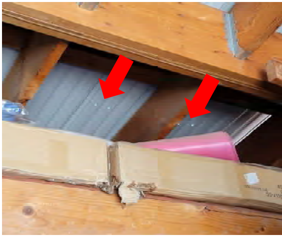
E3.1 Exposed Ceiling
