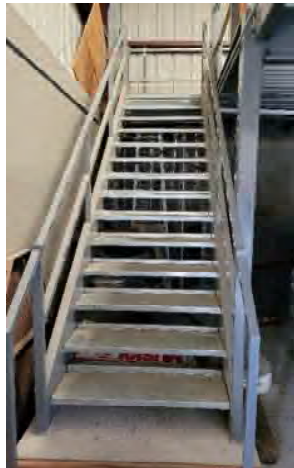
E7.1 Metal Stairs & Mezzanine
