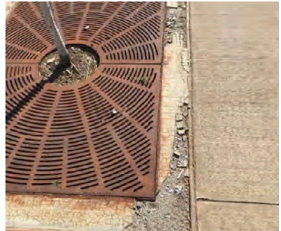
B5.1 Failing concrete at tree grates
