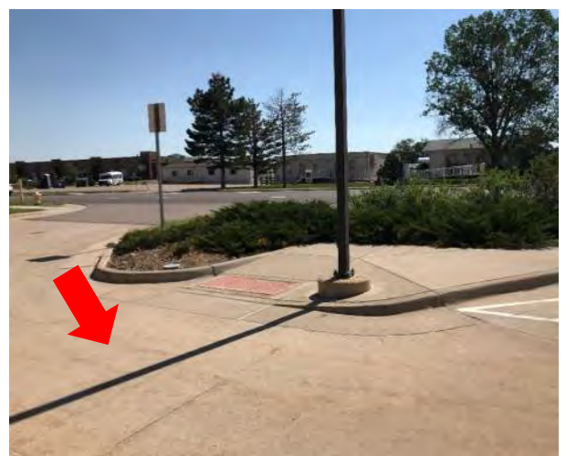
B7.1 Crosswalk across drive aisle at east entry recommended
