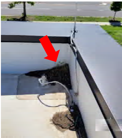
D1.3 Debris on Roof
