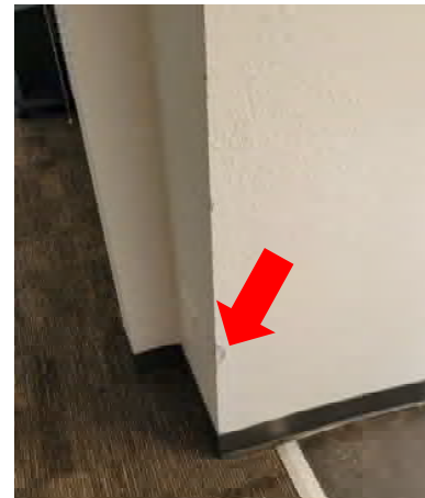
E2.1 Gypsum Board Walls
