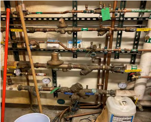
F1.1 Domestic Water Entry Backflow Prevention
