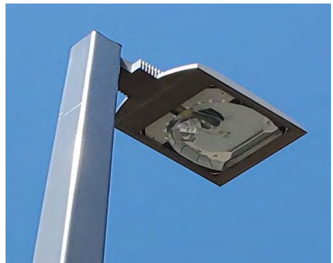
G3.1 Exterior Metal Halide Pole Mount Fixture
