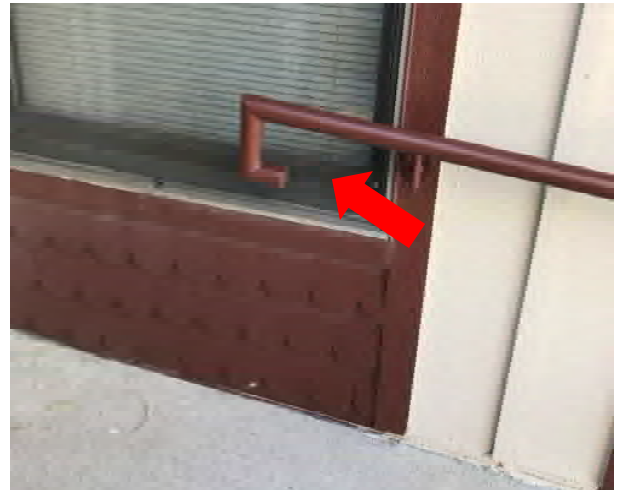
B4.1 Handrail should have full returns
