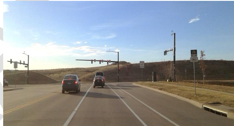
Figure 6 - View of the Chambers and Hess Road Intersection looking south.
