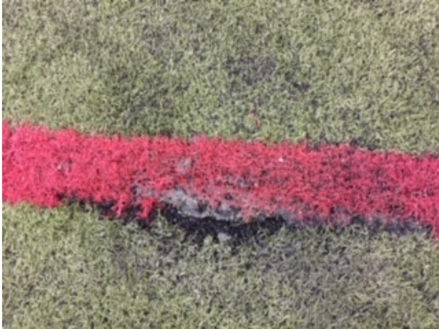
Shows a damaged seam that has been repaired multiple times.
