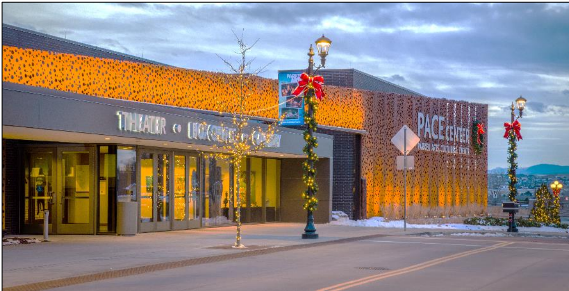
Figure 70 - The PACE Center building composition exhibits a variation in the top, middle and base requirement for horizontal massing breakdown, which meets the Design Standards. (Photo by: John Ott)
