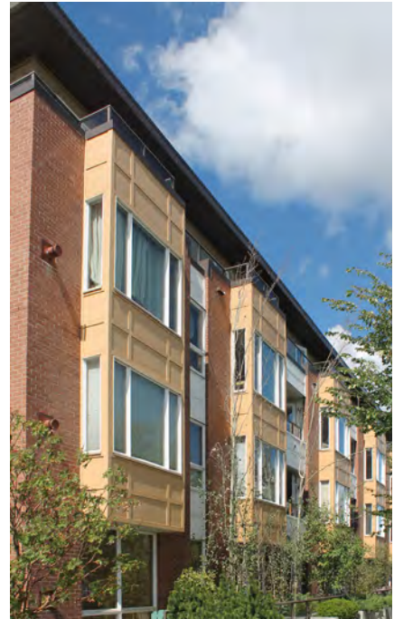
Figure 2.2 Example of Multiple-Family building
