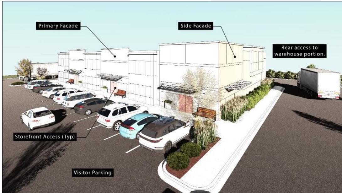
Figure 93 - Multi-tenant/flex office industrial building with warehouse and loading docks in rear of the building.
