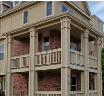
Figure 2.126 High-quality and well-designed wrapping Porch and Balcony
