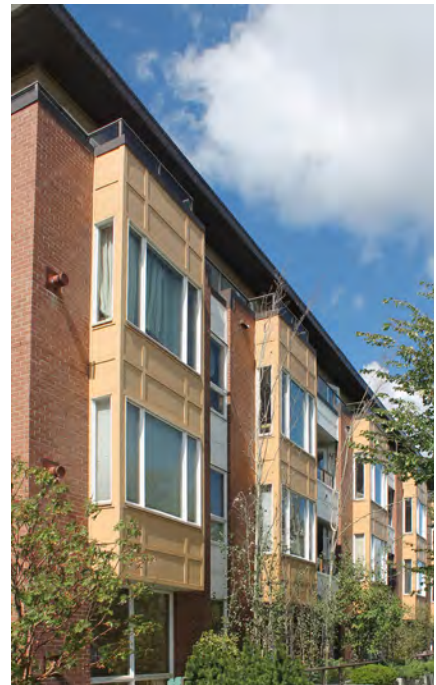
Figure 2.2 Example of Multiple-Family building
