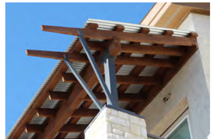
Figure 2.143 High-quality material (wood) used for exposed rafters of an awning
