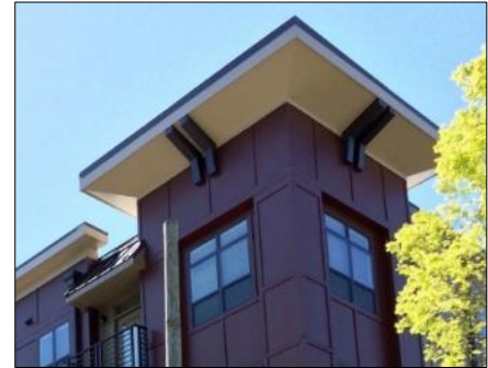
Figure 75 - Example of a large eave overhang.
