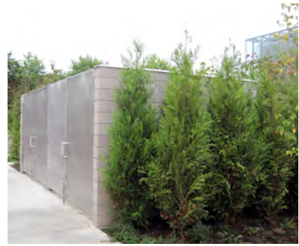
Figure 2.56 Screened outdoor storage
