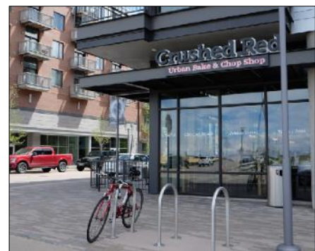
Figure 11 - Example of a mixed-use development
