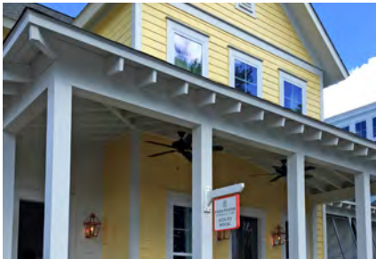
Figure 2.128 Simple Eave Overhang
