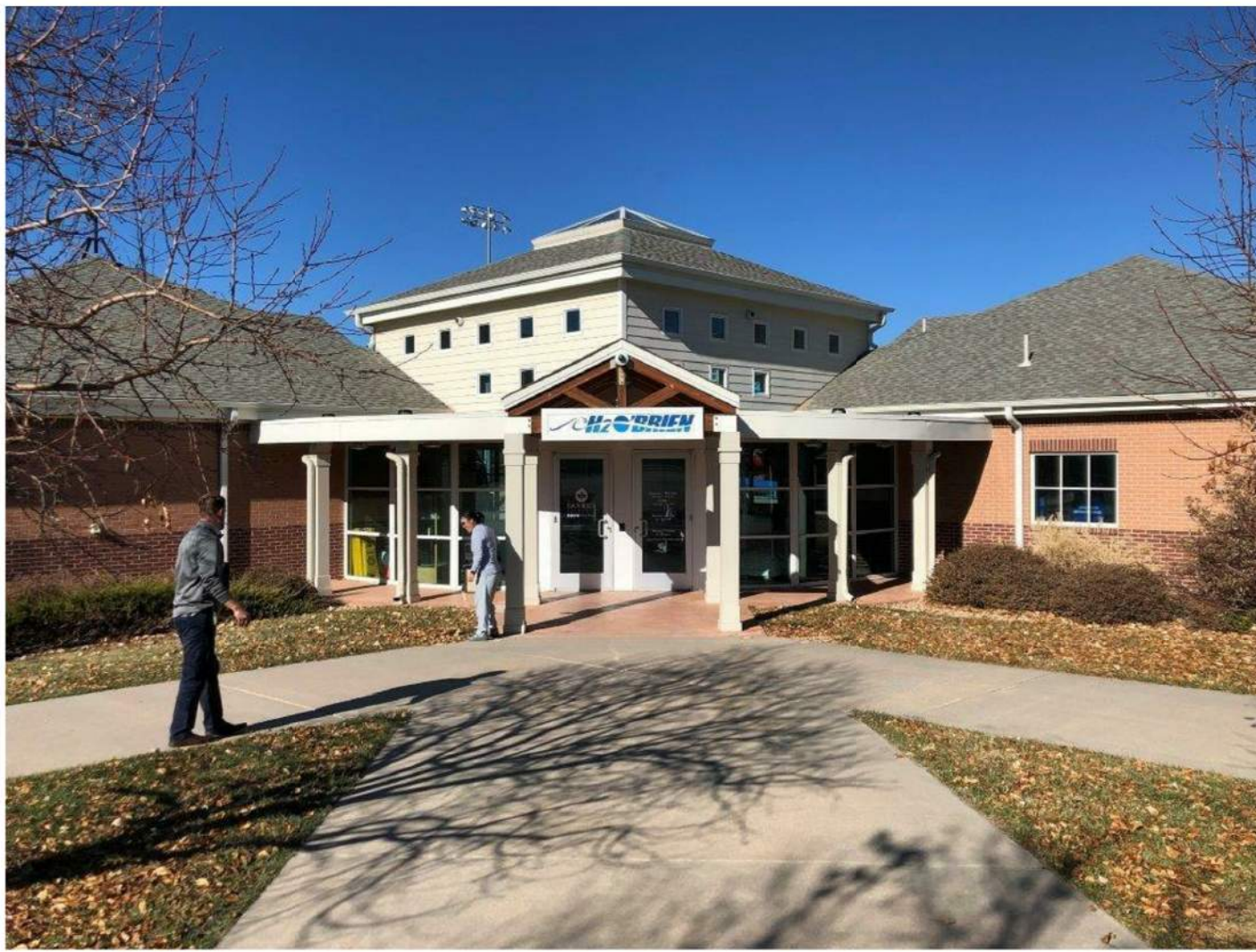
MAIN ENTRY - NO CHANGES TO EXISTING ELEVATION
