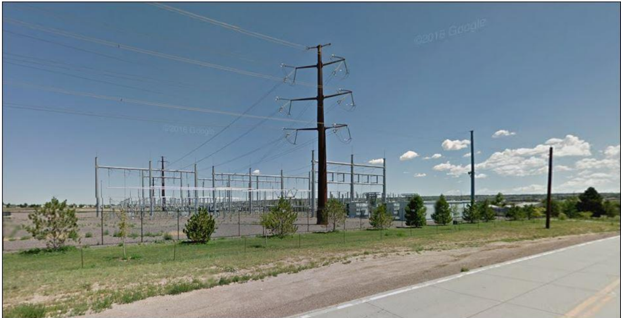
Figure 2 – View of Sulphur Substation, Looking Northeasterly
